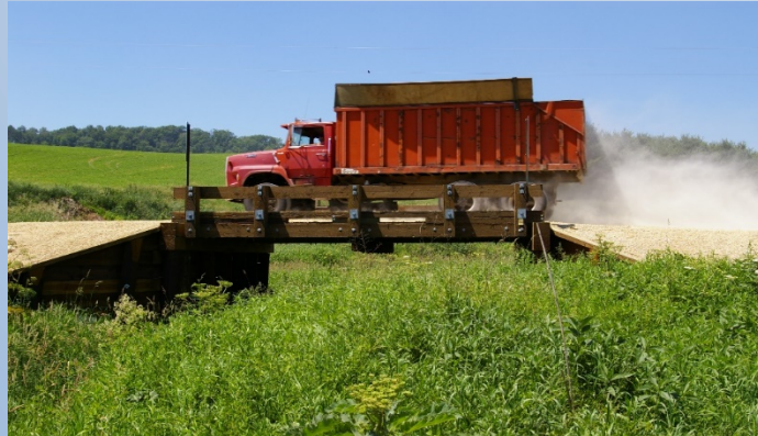
Timber Vehicle Bridge (Panel-Lam)
