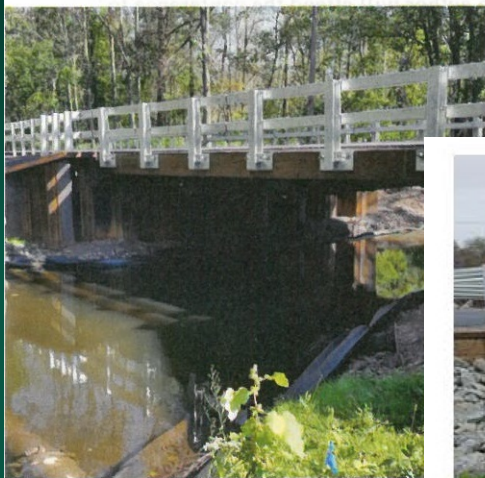
This is an example of an accelerated bridge construction utilizing perma steel sheet piles supplied by Skyline
