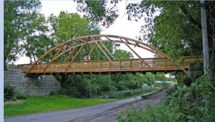
Timber Recreation Bridges
