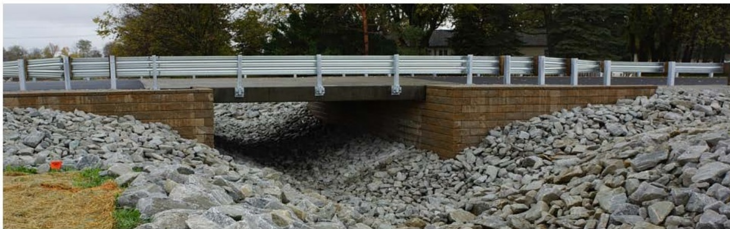
This is an example of an accelerated bridge construction utilizing perma steel sheet piles supplied by Skyline
