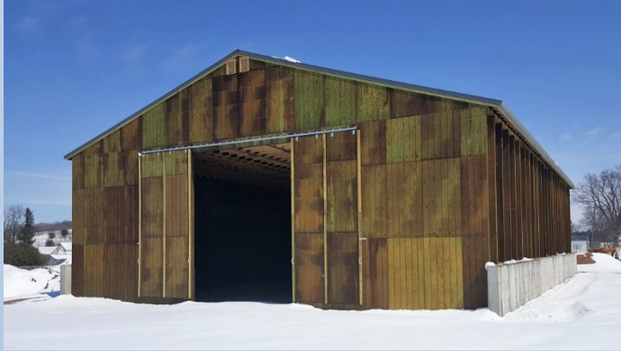
Salt Storage Buildings
