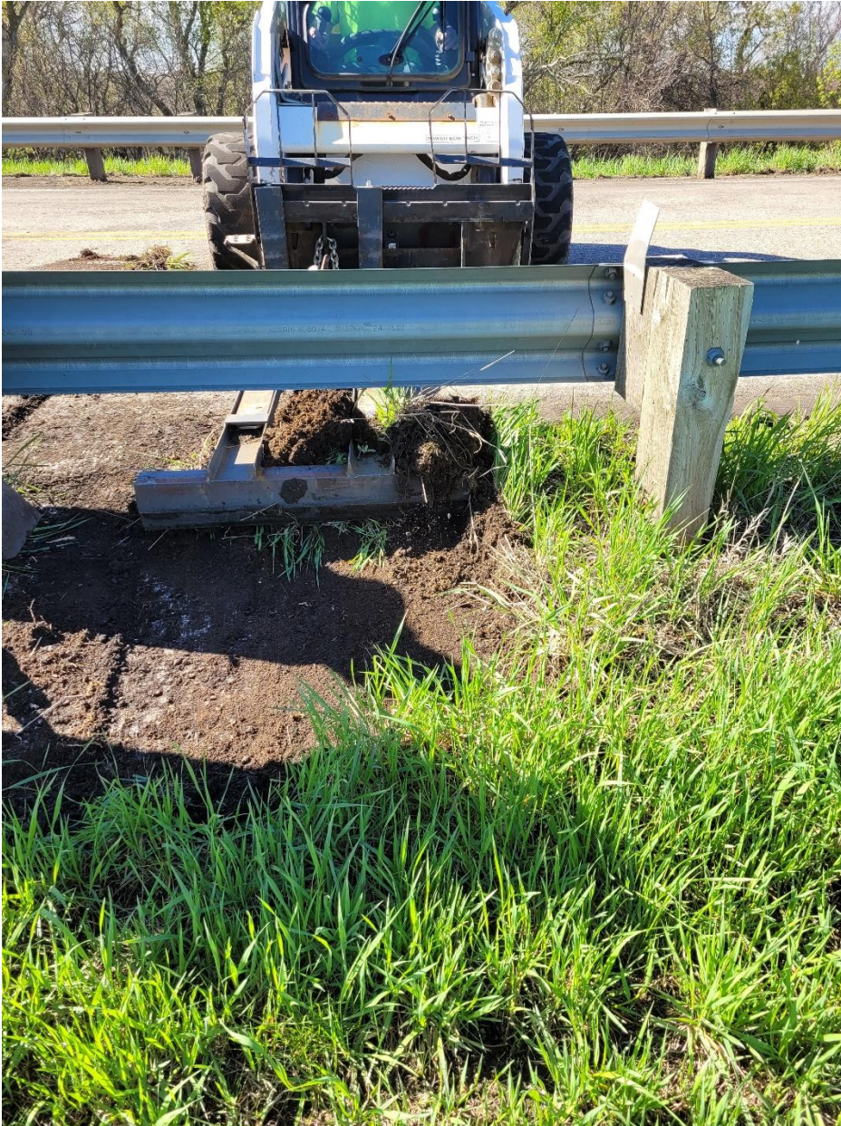
Bridge cleaner pulling the vegetation.
