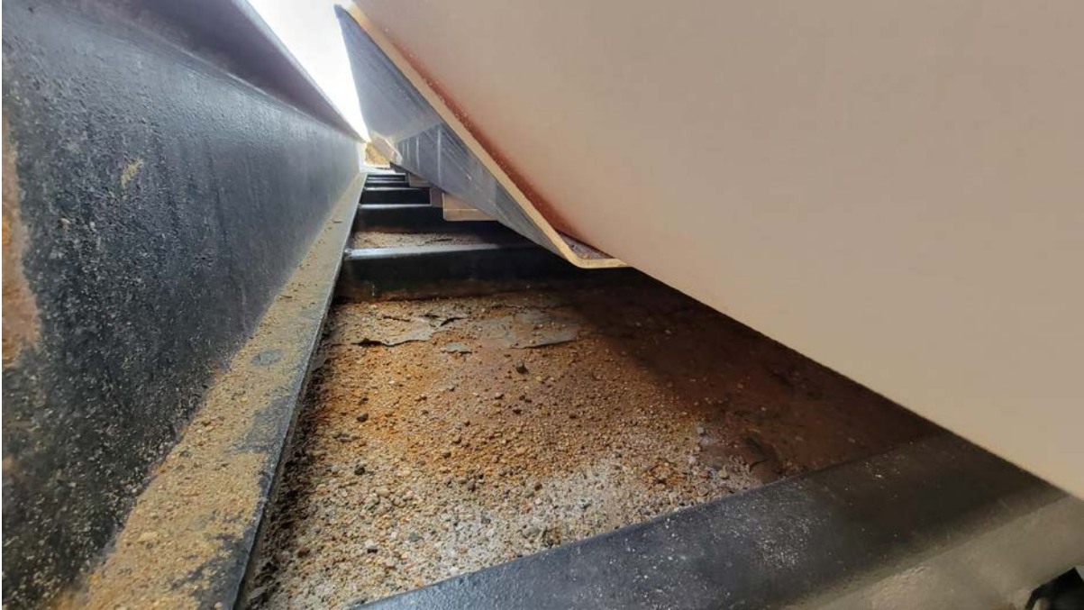
Cross beams for strength.
