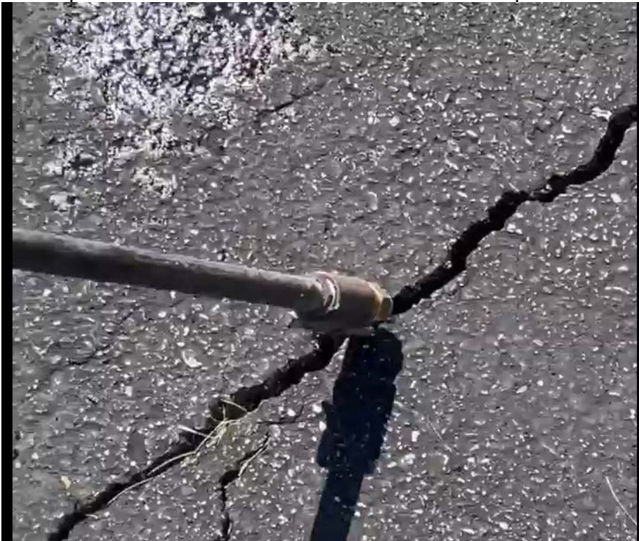
The asphalt crevice blaster is attached to an air compressor
