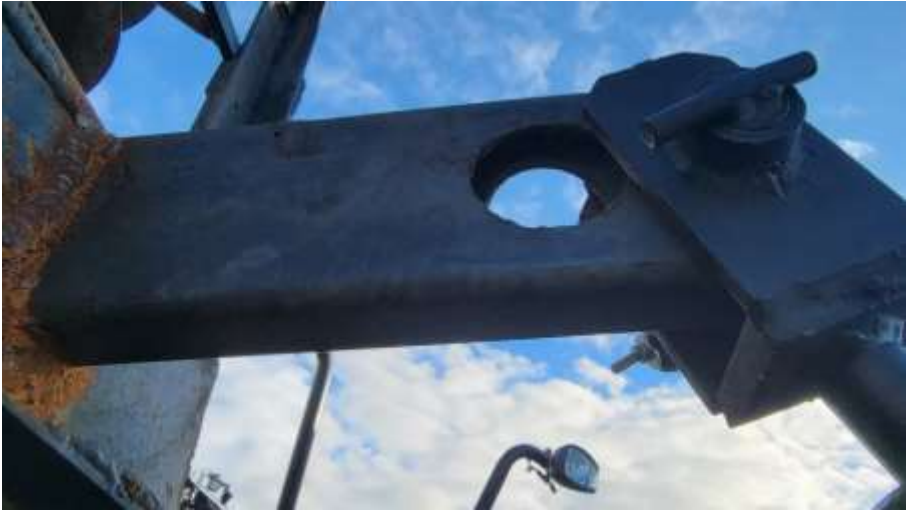
Tower for hydraulic cylinder
