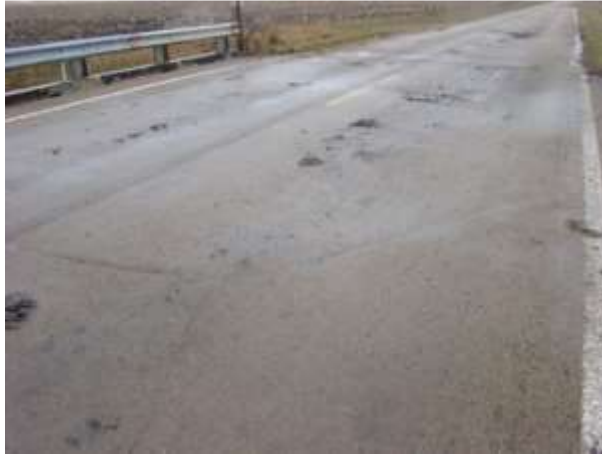
(a) Asphalt Overlay
