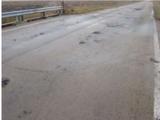
(a) Asphalt Overlay
