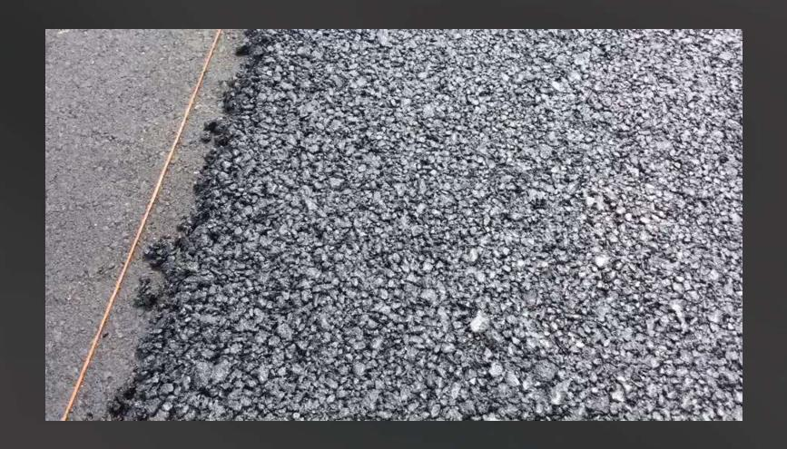
Edge Density between 88.0 and 88.9 on 4 tests
