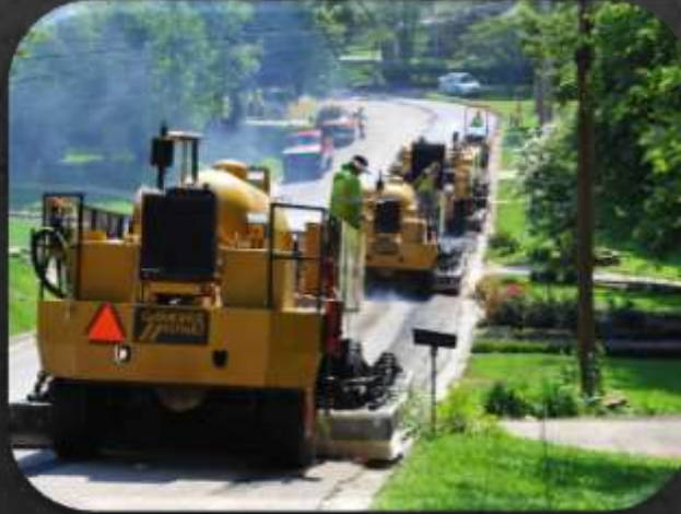
Soil Stabilization/ Modification
