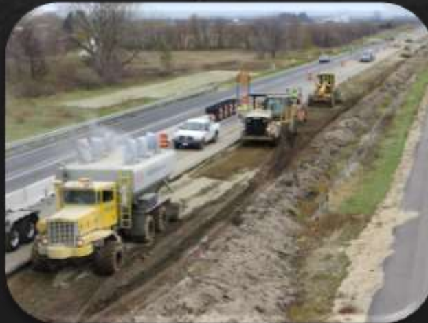
Soil Stabilization/ Modification
